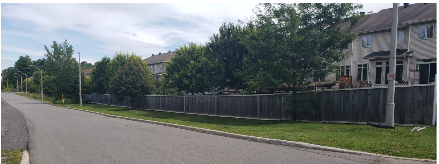
A ditch on the south side of Watters Road
