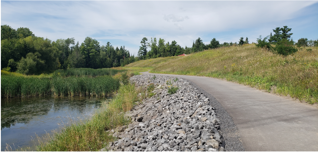
Possible slope stabilization with more vegetation cover
